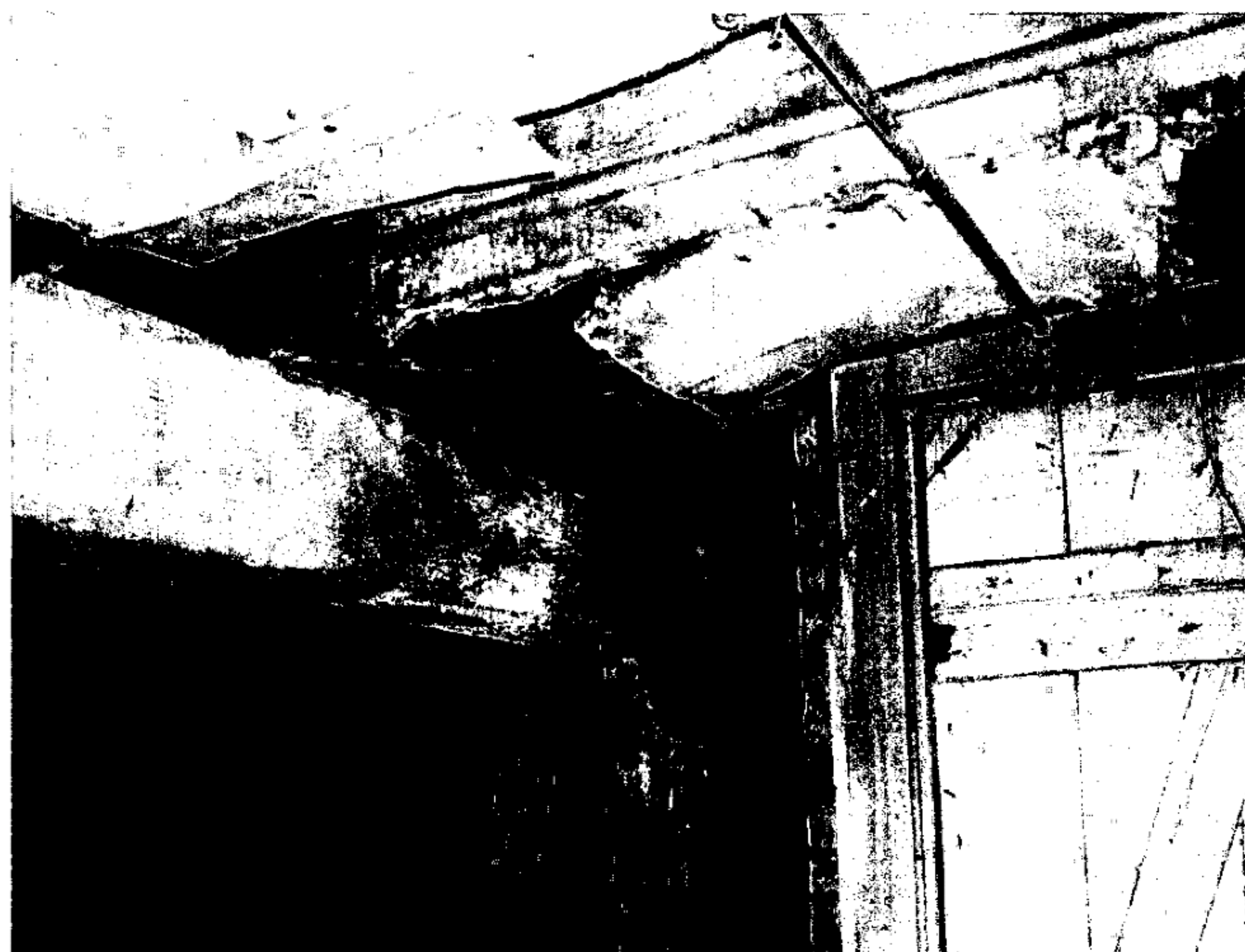
Photo No. 07 – Further Timber Column and Girder Support Settlement of 618 Atlantic Avenue (Condition on November 01, 2005)
