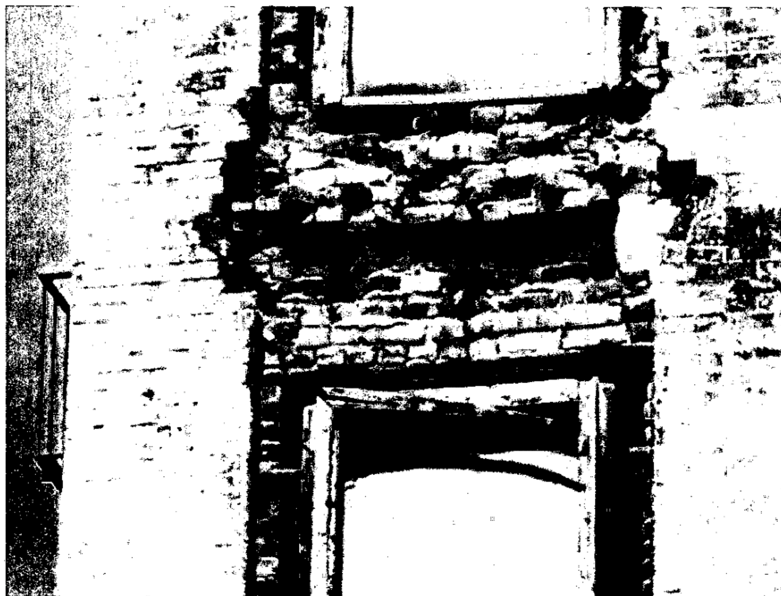
Photo No. 03 – Masonry East Bearing Wall Damage at 3 rd & 4 th Floors of 620 Atlantic Avenue
