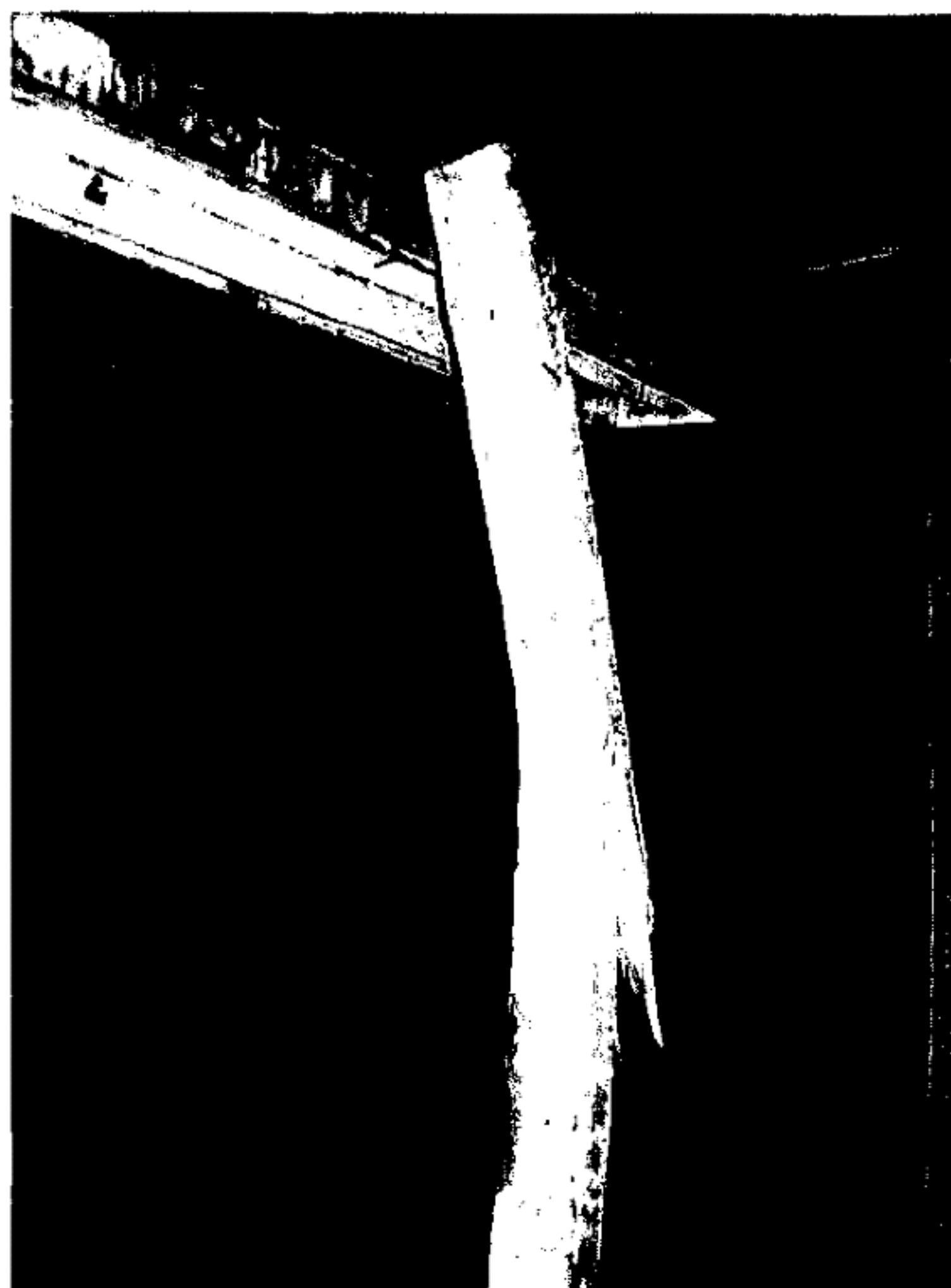
Photo No. 13 – Timber Post Failure At Basement of 461 Dean Street
